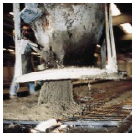
Casting slab with concrete admixed with MAPEFLUID IF328
