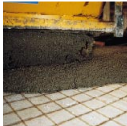
Pouring concrete admixed with MAPEFLUID IF328 for precast concrete panel
