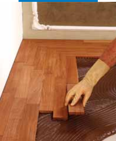
Installing a 14 mm Teak plank
