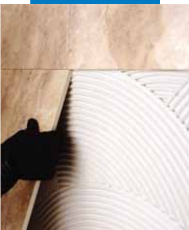
Laying large-sized porcelain tiles on walls
