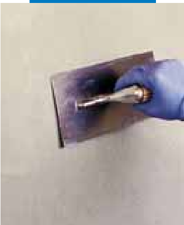
Smoothing Planitop 560 surface with a metal trowel
