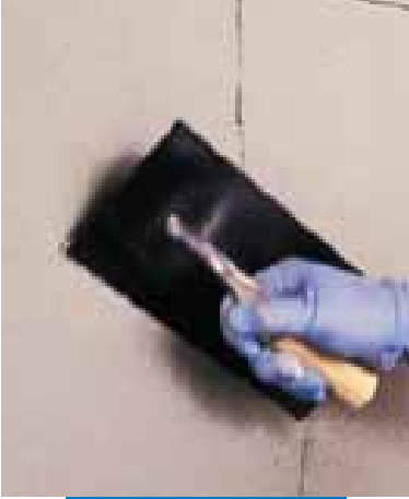
Applying Planitop 560 with a metal trowel
