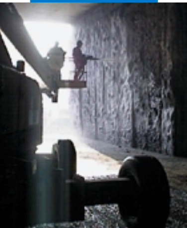
Spray application of mortar admixed with Mapeplast SF
