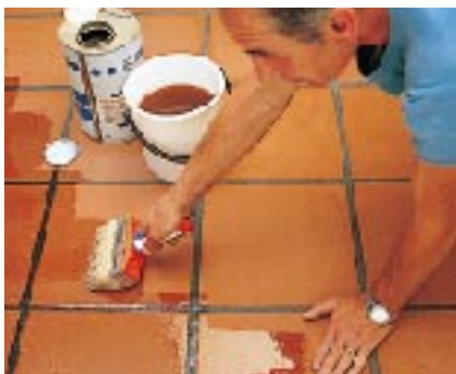
Spreading with a brush
