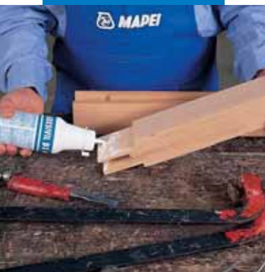
Bonding wood window frames for exteriors
