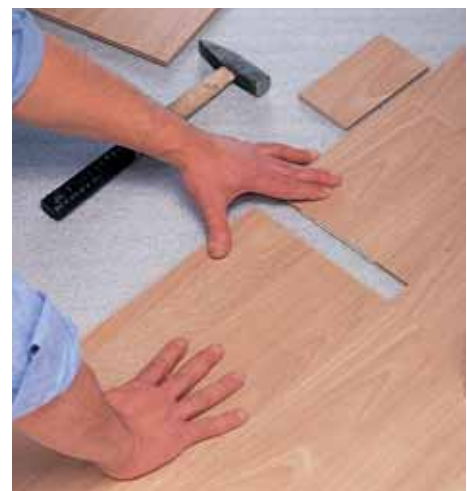
Placing tongue-and-groove sections of laminate flooring
